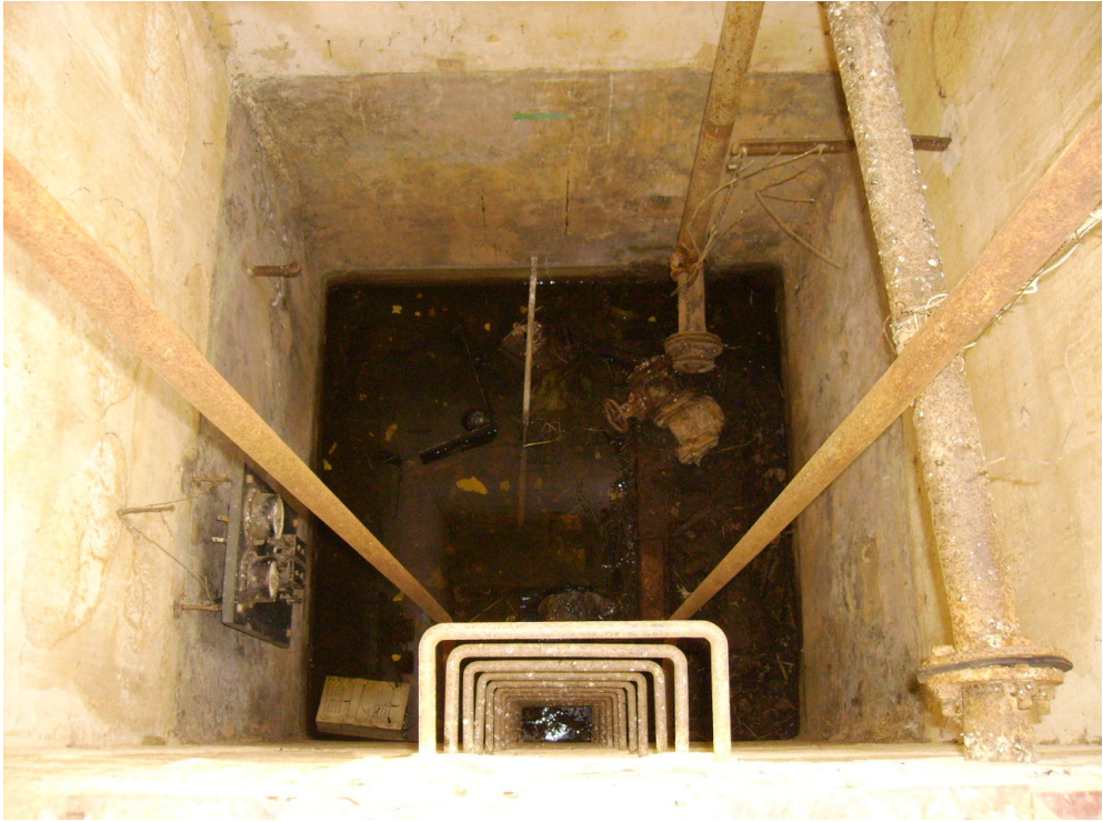
Interior caseta sondeo Villanueva
